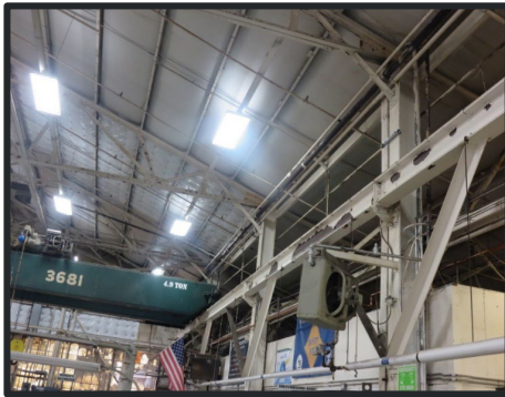
Temporary bracket located in crane travel path
