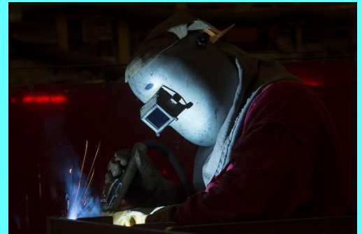
Shipbuilder Bobby Vaughan welds on a fixture for the Aircraft Carrier JOHN F KENNEDY CVN 79.
