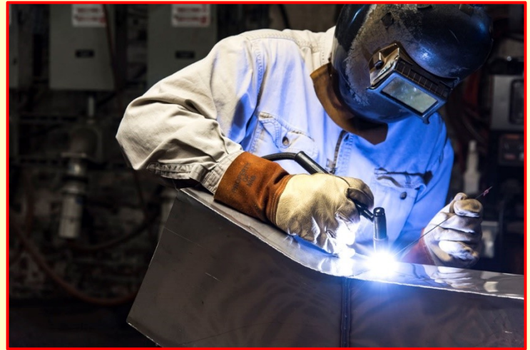
Shipbuilder welding in Building 205. Photo by Ashley Major.
