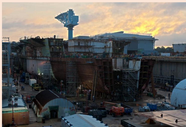
USS GERALD R. FORD (CVN 78) under construction. Photo by Rick Thompson
