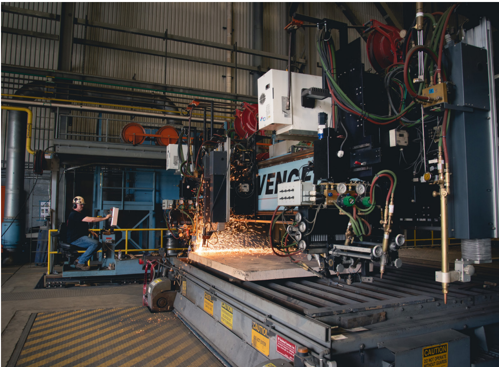
Gerald Bish prepares for the ceremonial first cut of steel for Doris Miller (CVN 81). Photo by Ashley Cowan
