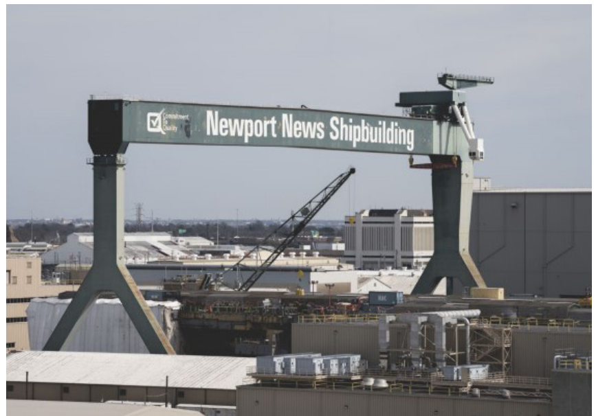
This 2018 photo shows the crane during the dry dock portion of USS George Washington 's (CVN 73) refueling and complex overhaul (RCOH). Photo by Matt Hildreth
