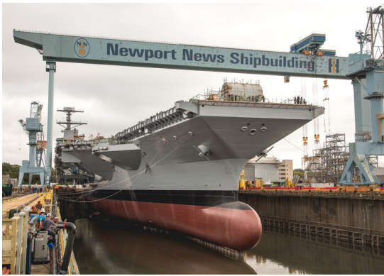
Water begins to fill Dry Dock 12. Photo by Ashley Cowan
