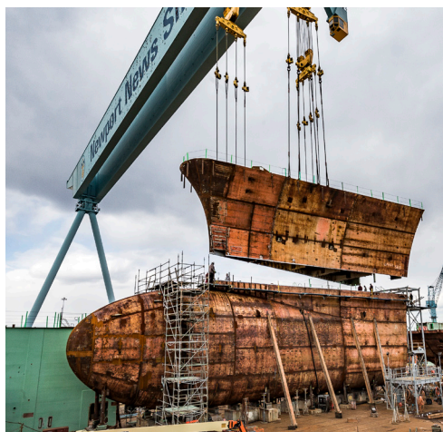
Shipbuilders recently completed a 260-metric-ton lift to connect the upper part of John F. Kennedy's lower bow Photo by John Whalen
