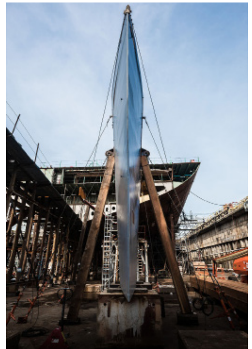
John F. Kennedy's (CVN 79) rudders await in dry dock. Photo by Matt Hildreth
