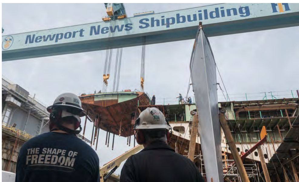
Cover photo: John F. Kennedy's (CVN 79) 932-metric ton lower stern was lifted into place June 22. Photo by John Whalen ; Pictured above: Shipbuilders watch as Kennedy's lower stern is lifted into dry dock. Photo by Matt Hildreth
