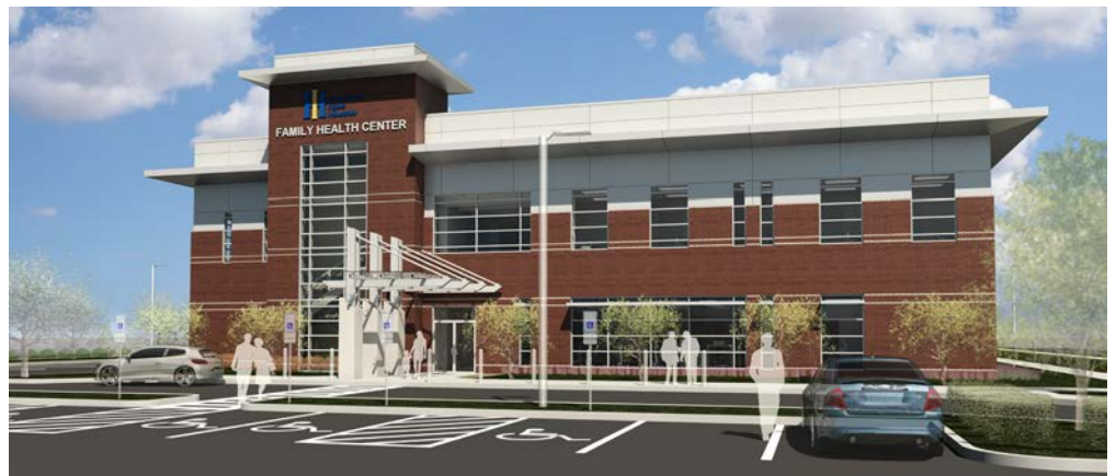
Photo illustration of the 21,894-square foot HII Family Health Center that is scheduled to open later this year.
