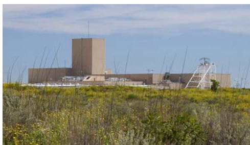
The Waste Isolation Pilot Plant (WIPP) in Carlsbad, New Mexico.
